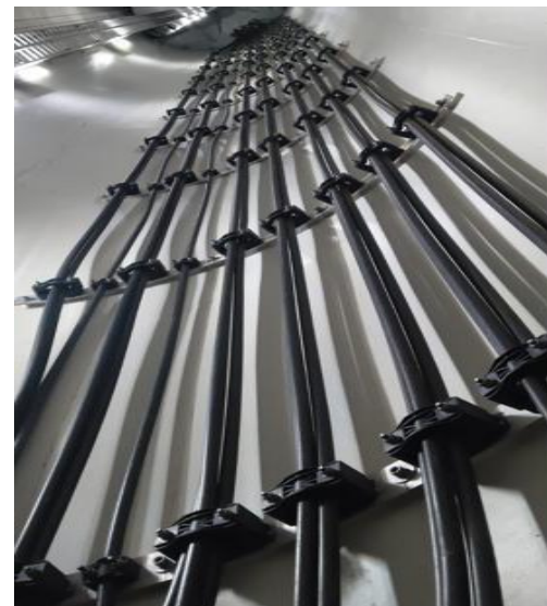
Figure 25: Cables arrangement after the retrofit
