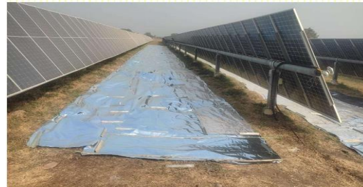
Figure 11: Reflective sheet installation on surface 4
