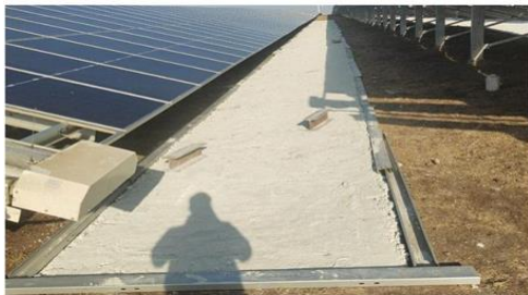
Figure 10: Preparation of surface for improving the albedo 3
