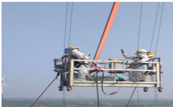
Figure 26: Team during WT blade cleaning
