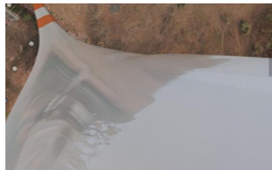
Figure 27: After cleaning the blade
