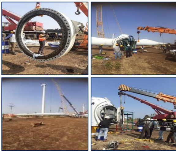
Figure 31: Replacement with Crane
